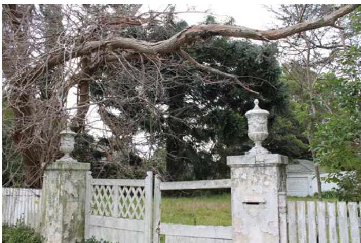
Figure 3.9 Fox Valley Road Original gates to 35 Fox Valley Road, Rothiemay
