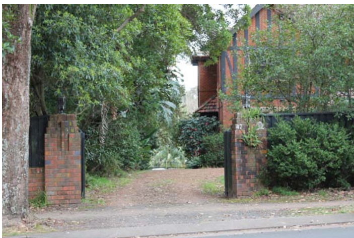
Figure 3.8 Fox Valley Road Original gate posts at 47 Fox Valley Road
